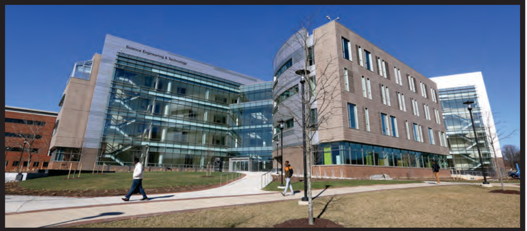
Science, Engineering and Technology Building at Howard Community College
